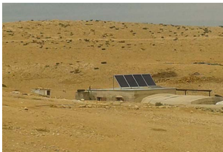
Solar panels in Arab Ar Rashaydeh
