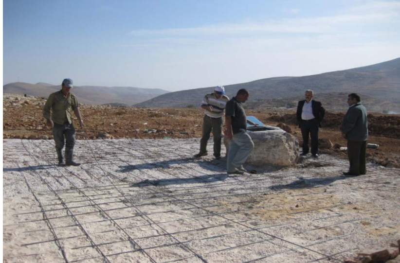
Works at one of the cisterns
