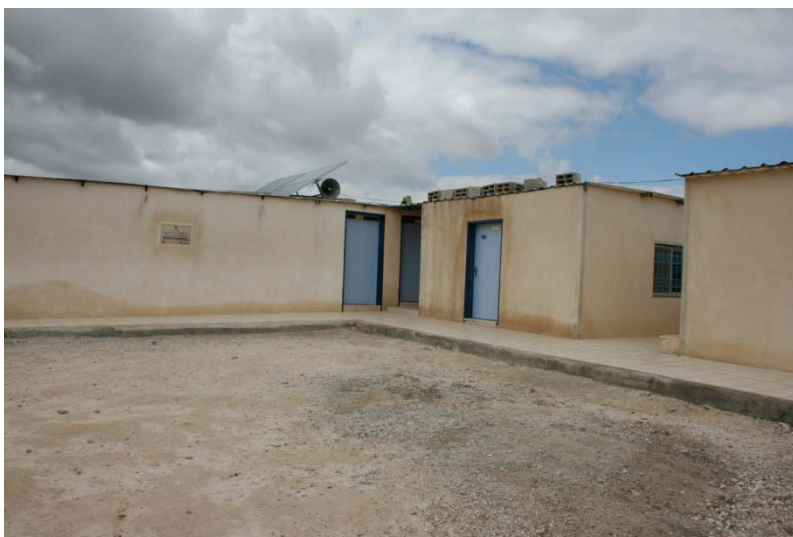
Renovation of Dkaika school
